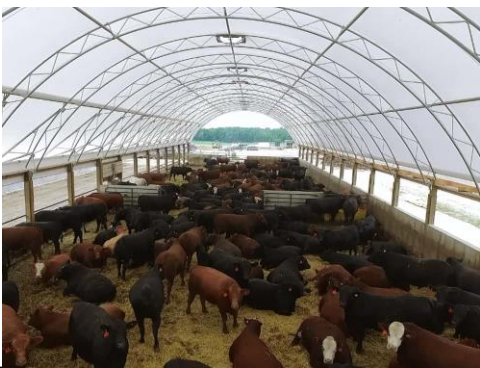
Example of a hoop building for livestock
