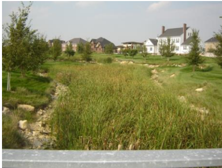
Example of a Drainageway or Surface Drain
