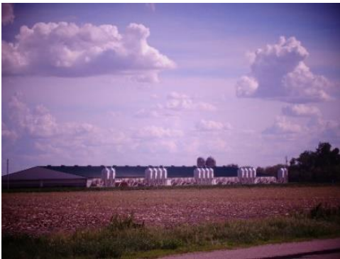
Example of an Animal Confinement Building
